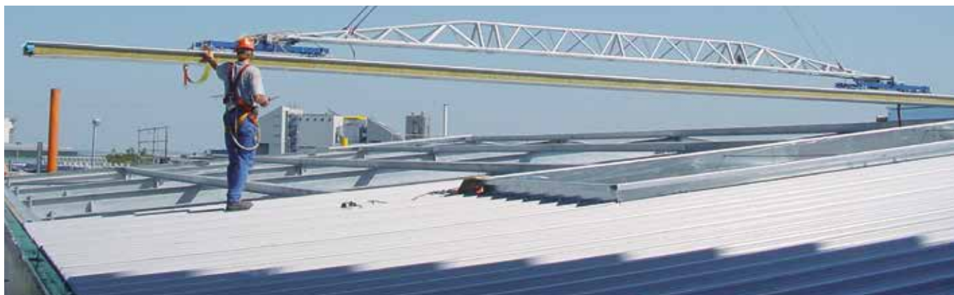
Example of roof assembly with traverse
