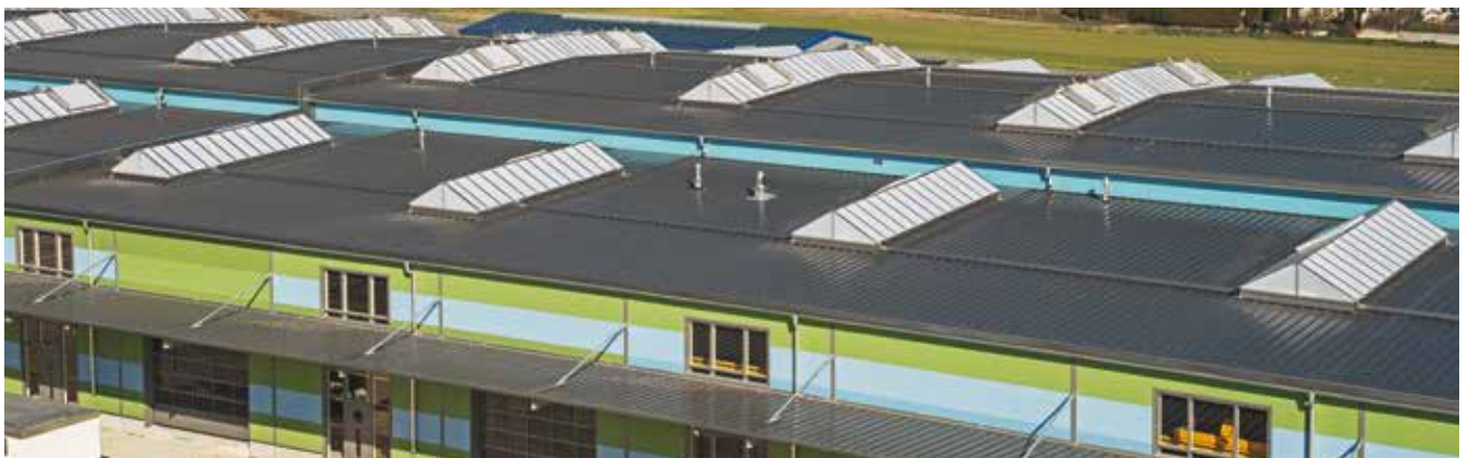
Production building with 24m roof panels
