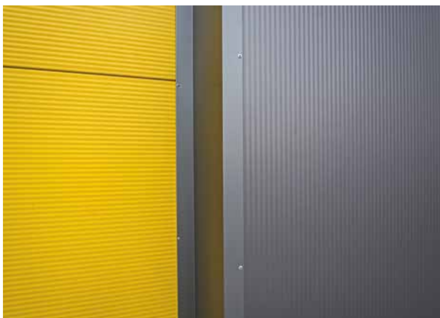
Horizontal and vertical laying
