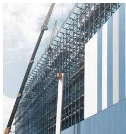
Special coating for use in maritime environments: Deep-freeze high-bay storage in warehouse in Grimbsby
